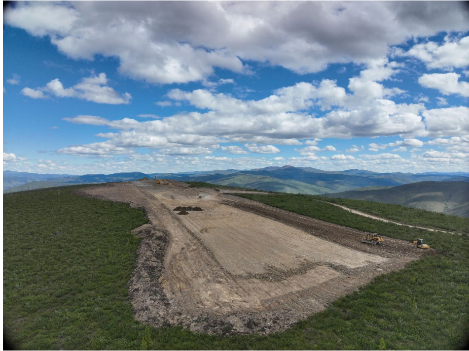
Figure 2. New airstrip under construction.
