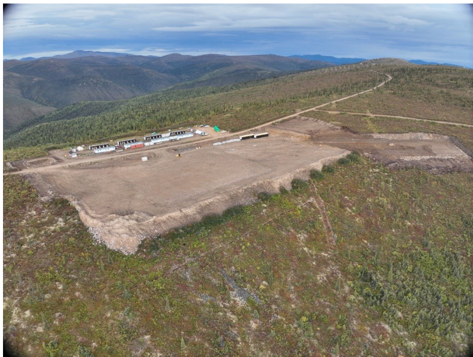
Figure 3. Construction Camp pad and initial modules.
